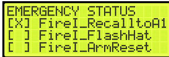
Figure 678: EMERGENCY STATUS Menu
