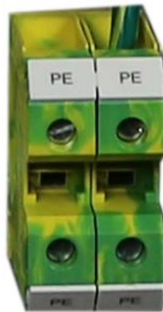
Figure 6: Ground Bus Terminal Blocks
