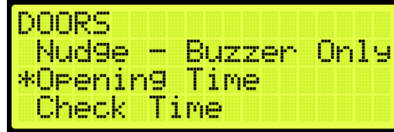
Figure 342: DOORS Menu – Opening Time
