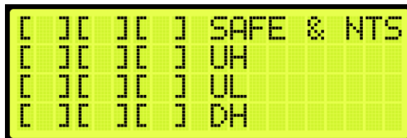
Figure 602: Valve Status Menu – Part 2 of 3
