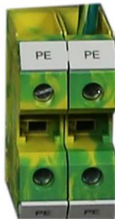
Figure 6: Ground Bus Terminal Blocks
