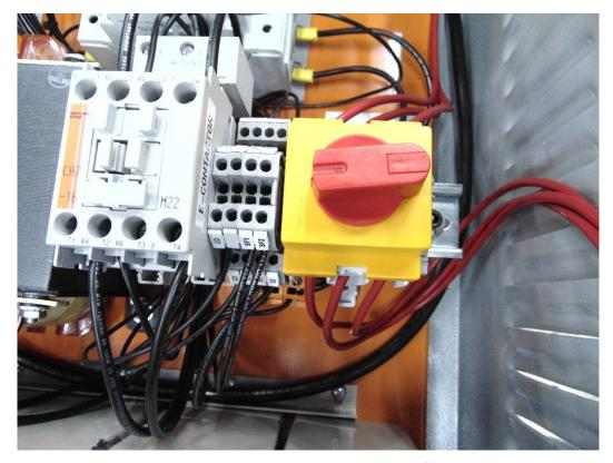
Figure 8: Battery Disconnect Switch - Off
