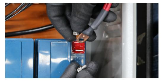
Figure 9: Remove Power and Ground Cable
