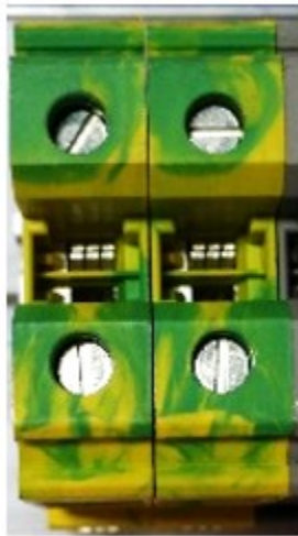
Figure 3: Ground Bus Terminal
